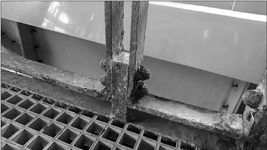
FIGURE 8.2 Rusty steelwork
